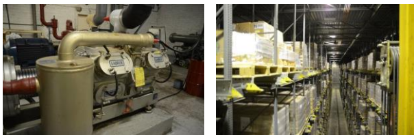
Figure 5. Compressor (left) used as a thermoelectric & vibrational ambient energy source. Indoor cold room lighting (250 Lux) also used as PV source for temperature & humidity sensors
